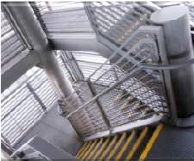
A steel staircase with colour-contrasted nosings provides an example of good stair design. The design would have been even more accessible for people with vision loss if colour contrast had been applied to the handrails.
